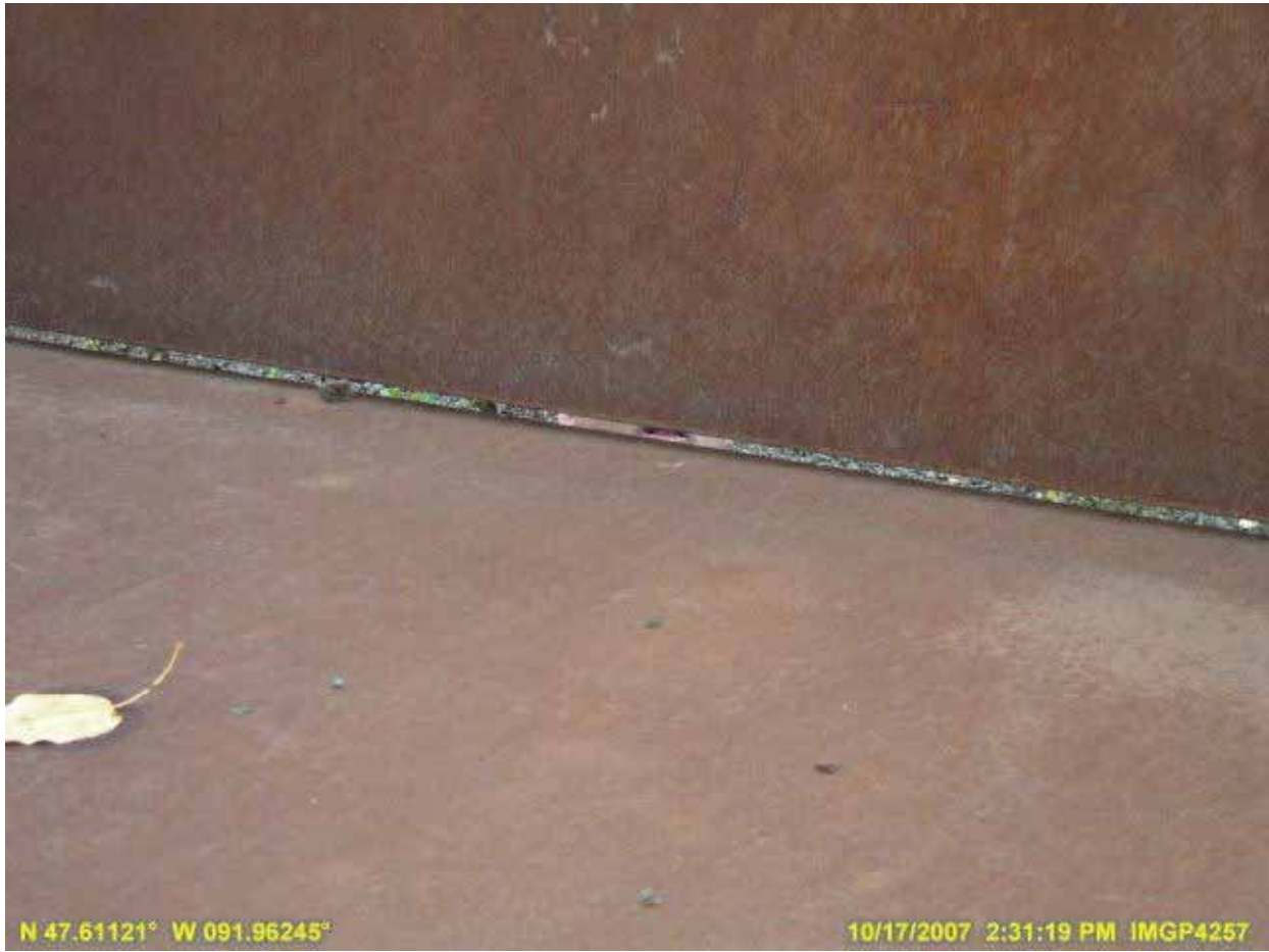
Figure 2. Gap in the side hinge of the rail car.
