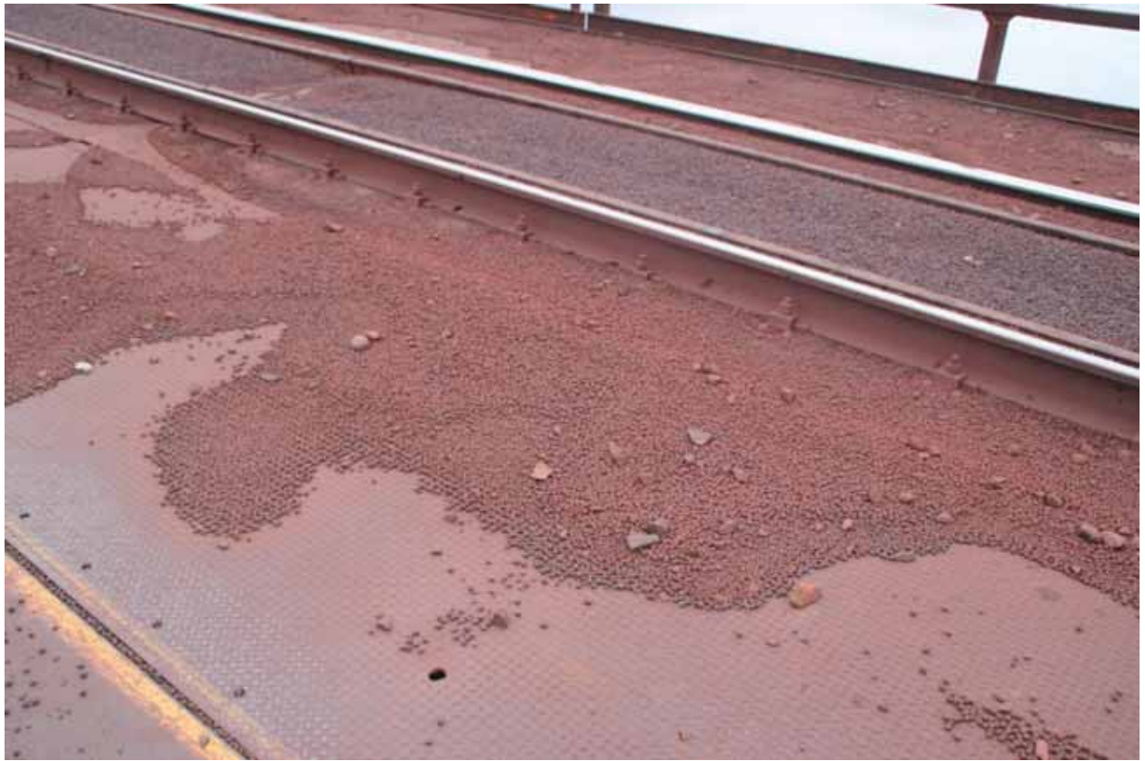
Figure 1. Spilled taconite pellets on a bridge above the Partridge River.
